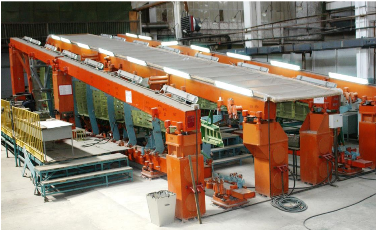
Fig 4.7. General View of Jigs and Fixtures for Assembly of Wing Torsion Boxes
